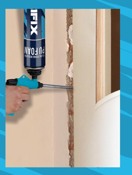
Fixing and insulating of door and window frames.
